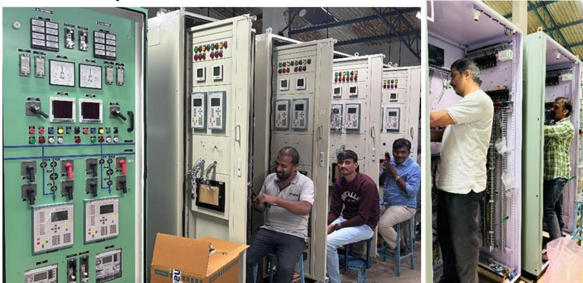
❖ Testing of Control & Relay Panels
